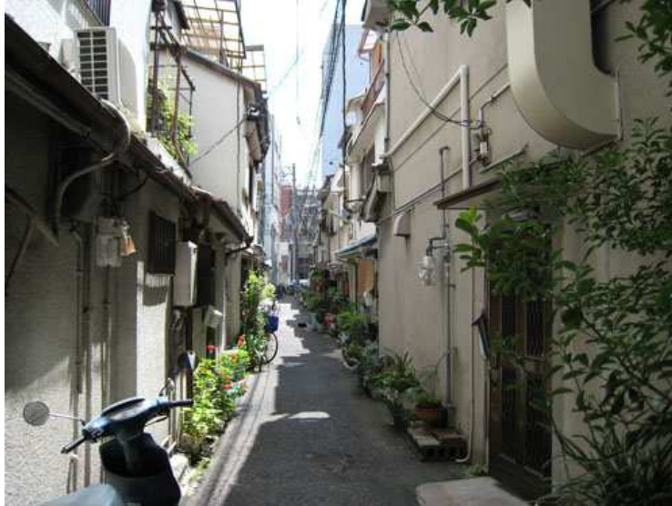
Figure 2.— Street view in a densely-built urban area.
